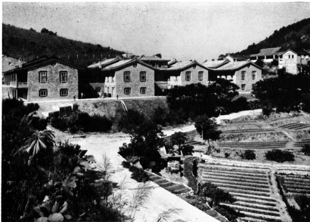
FIG. 4. Architectural appearance of Maxwell Memorial Medical Centre. Other buildings on Hay Ling Chau reflect the same general motif.
