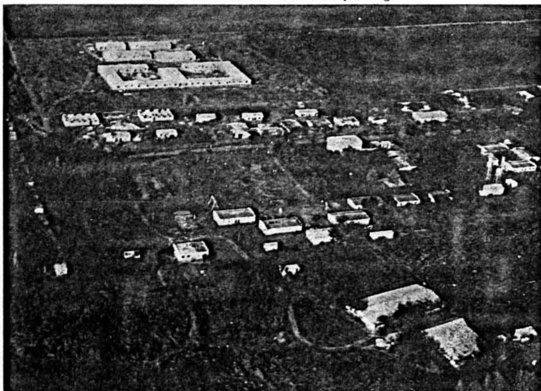
FIG. 2. Relief Center Bisidimo today. In the background the new building of the leprosy-clinic is seen.
